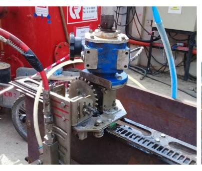
CR Asia Thailand (CRAT) was engaged by Shell Brunei to remove a partially collapsed storage tank roof. A total of 60 roof panels were removed using hydro abrasive cutting and CR Asia's patented track system.
